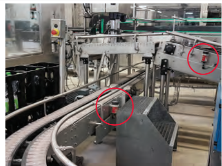
Chain lubrication on box transport system after packaging machine and full crate check
