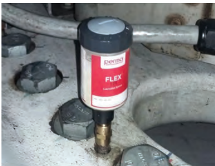
Yaw bearing lubrication
