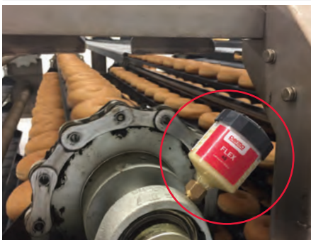
Lubrication of pillow block bearing on a cooling section for baked goods
