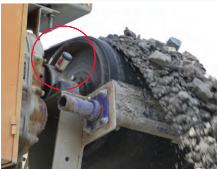
Lubrication of pillow block bearing on a conveyor
