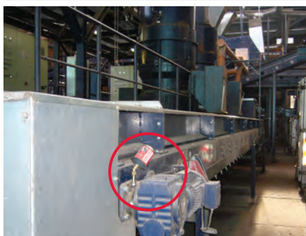
Flange bearing lubrication on a conveyor
